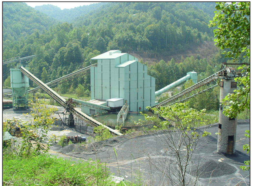
Among the many technological "fixes" that utilities are using to try to stave off global warming is "coal washing" to filter out impurities. Pictured here is a now-decommissioned coal washing facility located in Clay County, Eastern Kentucky. (Photo courtesy of Wikipedia)
